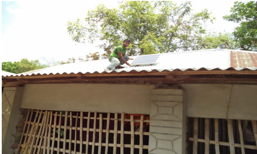
BASCO Foundation's staff is setting a solar panel.
